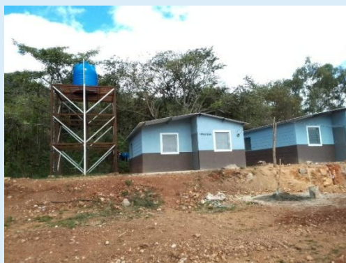
Photo 3 and 4. Safe Water Storage Tank and connections from the water source to each of the 15 homes.
